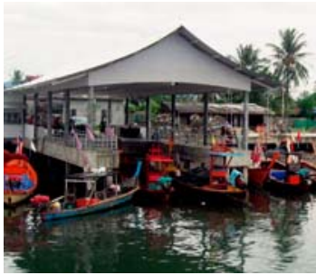
The Long-Tail Fishing Boat Repair Center and Pier
